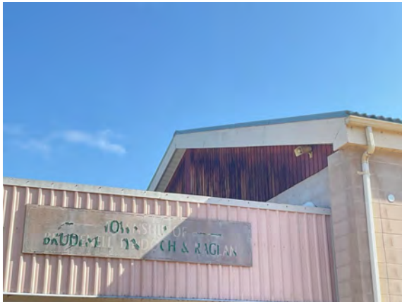
Quadville Public Works Garage - B201026
