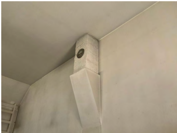
Palmer Storage Shed - C301005
