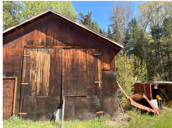
Storage Building - Quadeville - C102025
