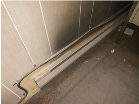
Palmer Public Works Garage - D305010
