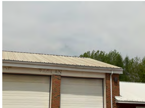
Palmer Public Works Garage - B301028
