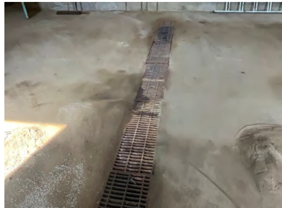
Quadville Public Works Garage - A103001
