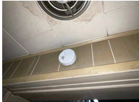
Palmer Public Works Garage - C301022
