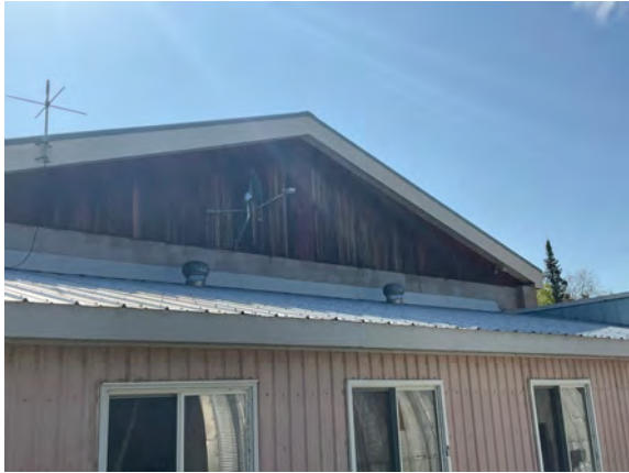
Quadville Public Works Garage - B201026
