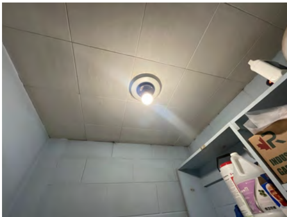
Quadville Public Works Garage - C303004
