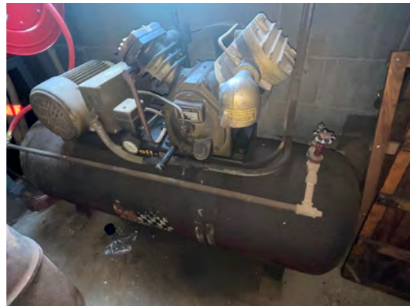
Palmer Public Works Garage - D209006
