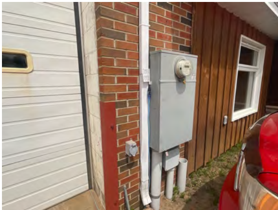
Palmer Public Works Garage - G401011
