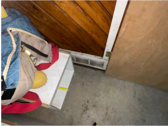
Brudenell Fire Hall #4 - D304001
