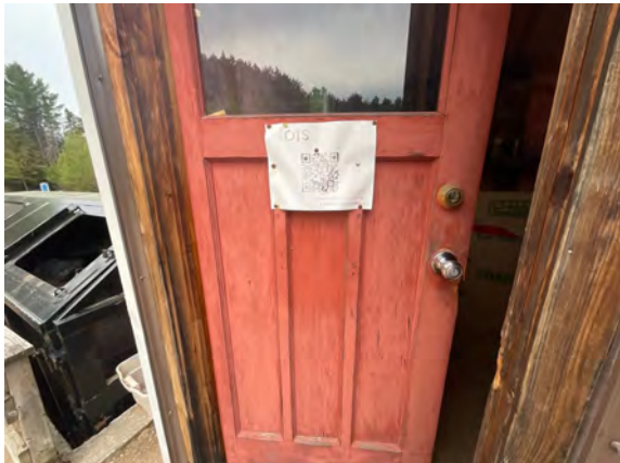
Raglan Transfer Station - C102022
