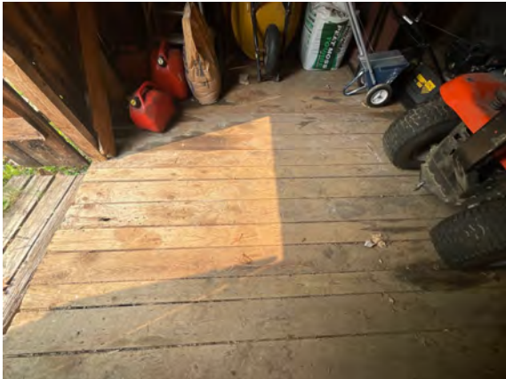
Four Season Park - Storage Building - A103001
