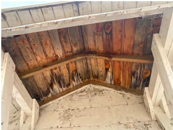
Palmer Fire Hall 1 - B201008
