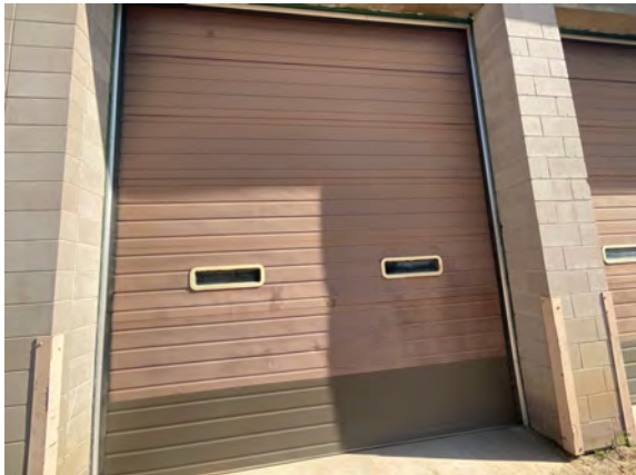
Quadville Public Works Garage - B203022
