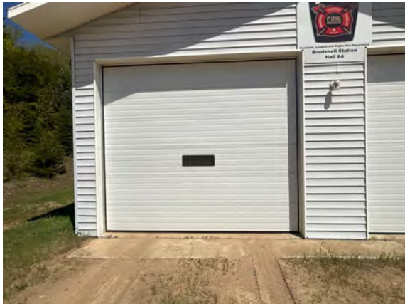
Brudenell Fire Hall #4 - B203022
