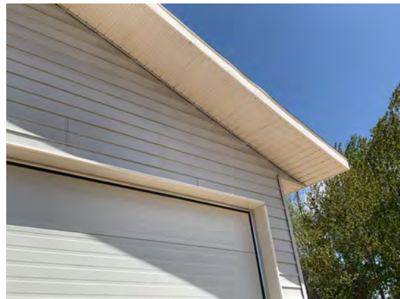
Brudenell Fire Hall #4 - B201008
