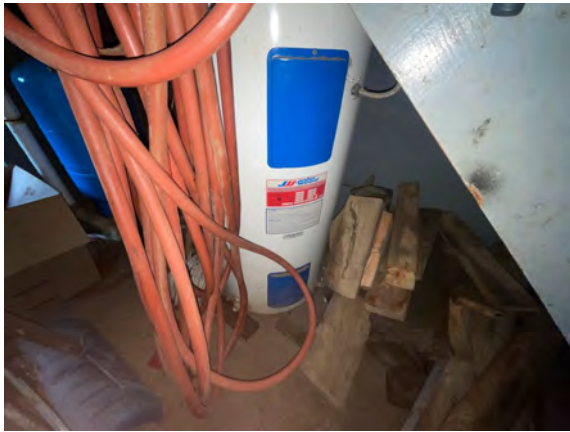
Palmer Public Works Garage - D202034
