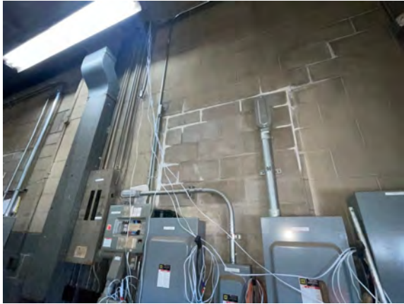
Palmer Public Works Garage - B103001
