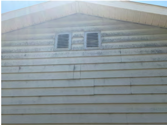
Brudenell Fire Hall #4 - B201005
