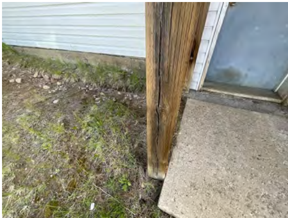
Quadville Fire Hall #3 - F101099
