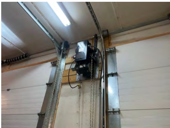
Brudenell Fire Hall #4 - B203022
