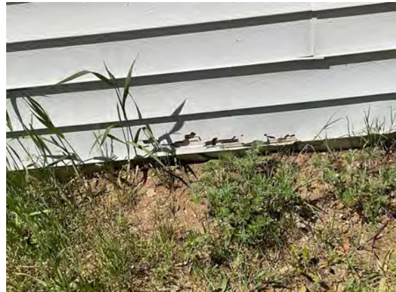
Brudenell Fire Hall #4 - B201025
