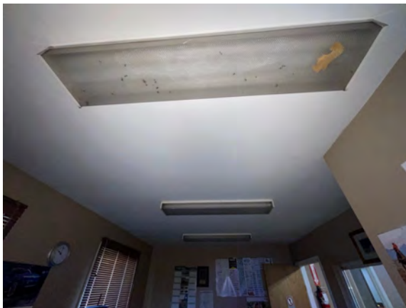
Quadville Public Works Garage - C303099
