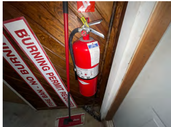
Brudenell Fire Hall #4 - D403002
