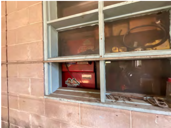
Quadville Public Works Garage - C101005
