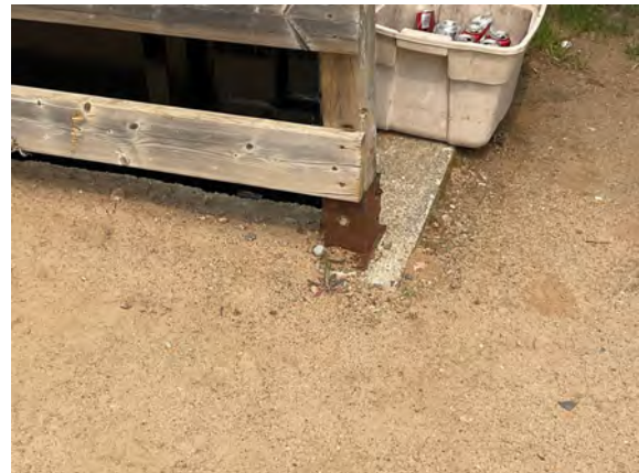
Raglan Transfer Station - A103001
