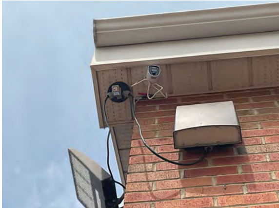
Palmer Public Works Garage - D502041
