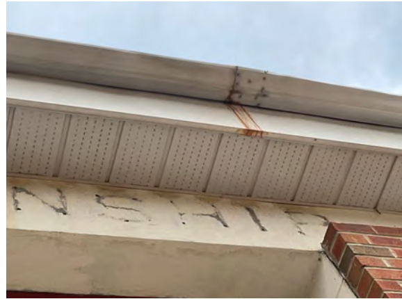
Palmer Public Works Garage - B201008
