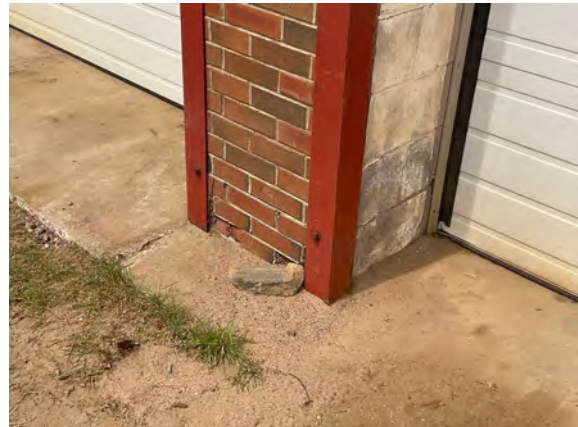
Palmer Public Works Garage - B201021
