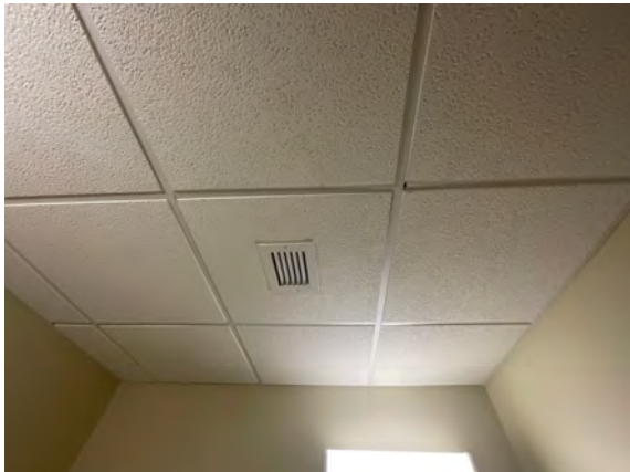
Township Office - D304033
