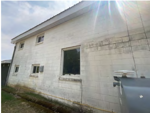
Palmer Public Works Garage - B201010
