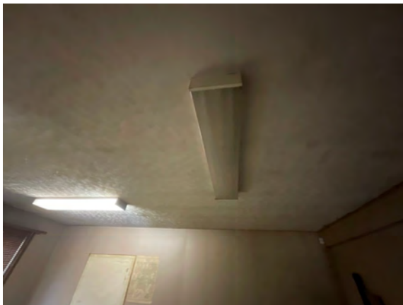
Quadville Public Works Garage - C303099
