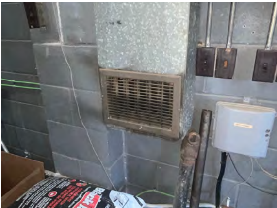
Palmer Public Works Garage - C303005
