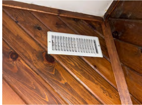
Brudenell Fire Hall #4 - D304001
