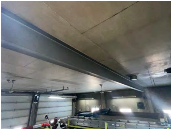
Palmer Public Works Garage - E103006
