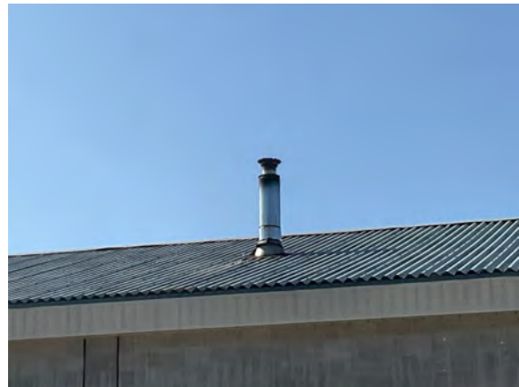
Quadville Public Works Garage - B301028
