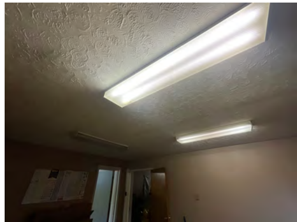
Quadville Public Works Garage - C303099
