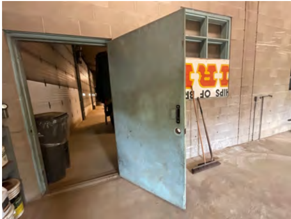
Quadville Public Works Garage - C102022
