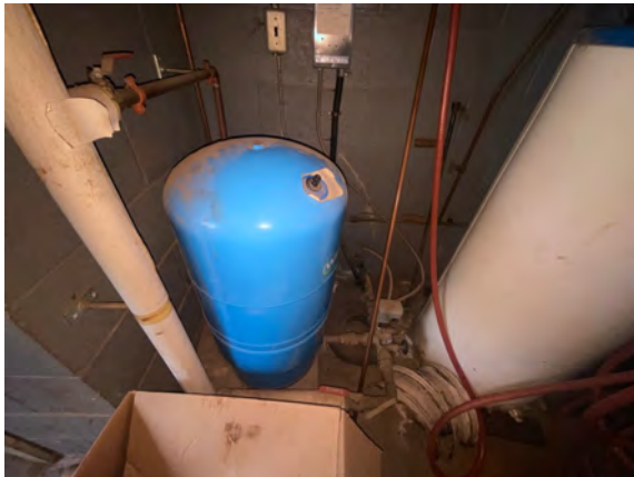
Palmer Public Works Garage - D202021
