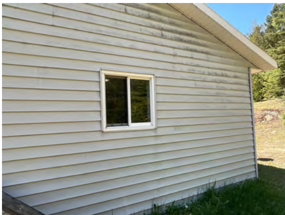
Brudenell Fire Hall #4 - B201025
