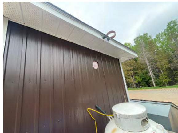
Raglan Transfer Station - B201024
