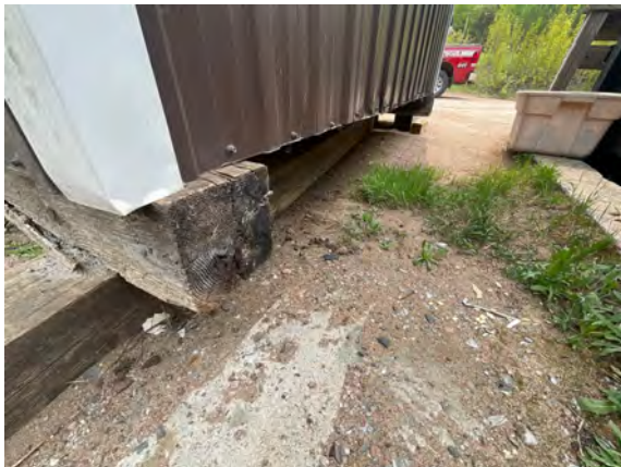
Raglan Transfer Station - A103001
