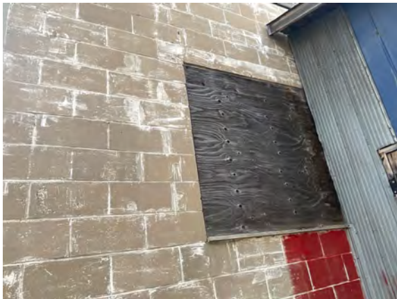
Palmer Fire Hall 1 - B201021
