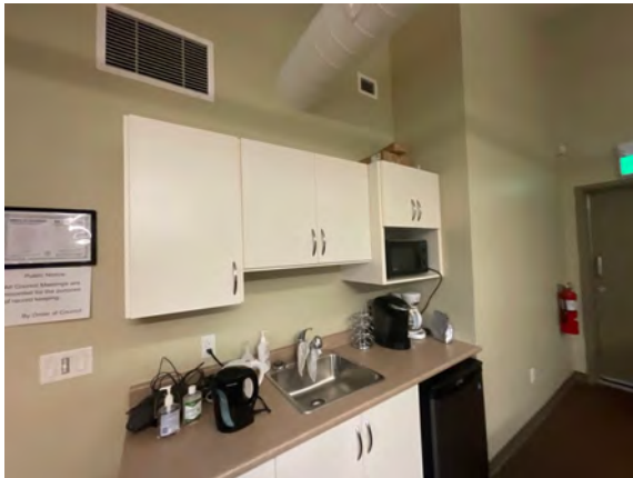
Township Office - C101001
