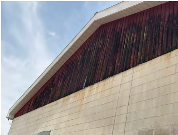
Palmer Public Works Garage - B201026
