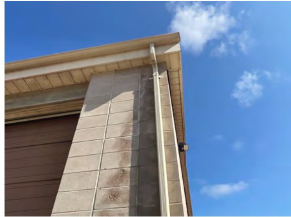
Quadville Public Works Garage - B301005
