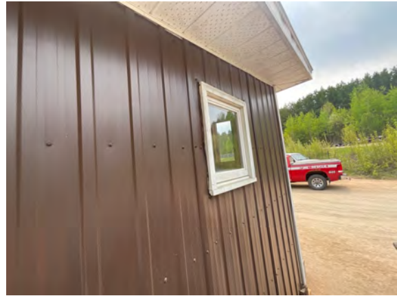
Raglan Transfer Station - B202001
