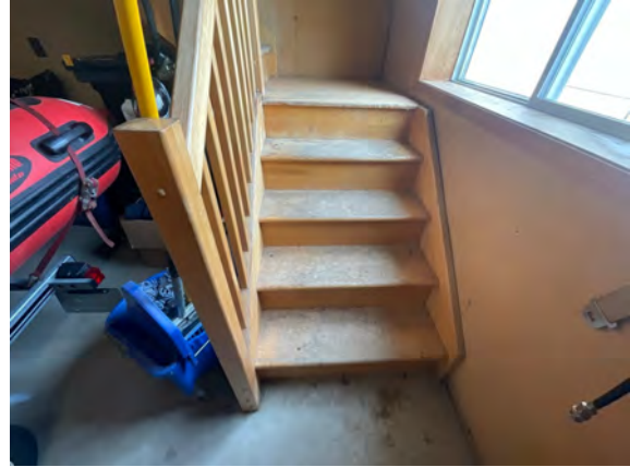
Palmer Fire Hall 1 - C201001
