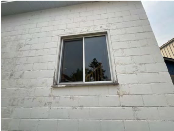
Palmer Fire Hall 1 - B202001
