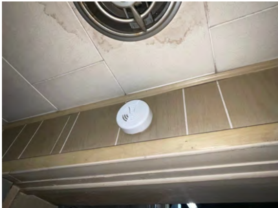
Palmer Public Works Garage - C303004
