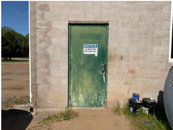
Quadville Public Works Garage - B203023
