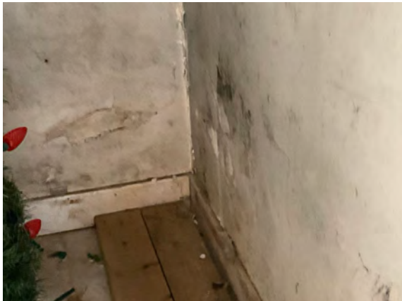
Palmer Storage Shed - C301022
