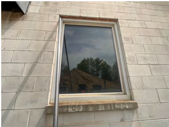
Palmer Public Works Garage - B202001
