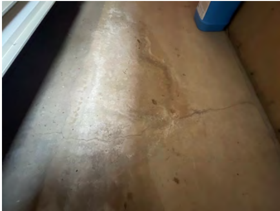
Palmer Fire Hall 1 - C302007
