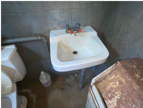
Palmer Public Works Garage - D201003
