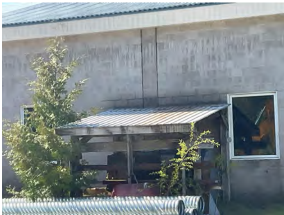
Quadville Public Works Garage - B201021
