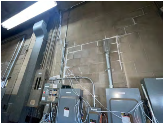
Palmer Public Works Garage - C101001
