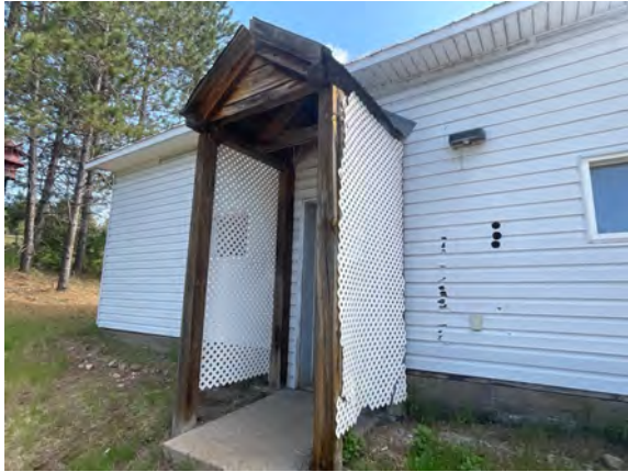
Quadville Fire Hall #3 - F101099
