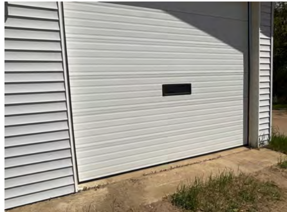
Brudenell Fire Hall #4 - B203022
