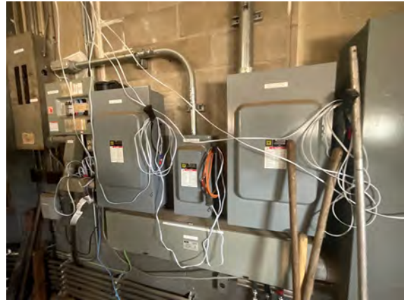
Palmer Public Works Garage - D501031
