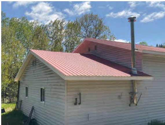
Brudenell Fire Hall #4 - B301028
