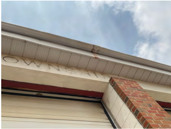
Palmer Public Works Garage - B201008
