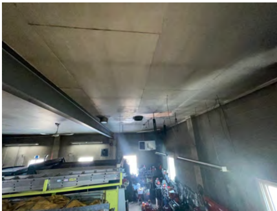
Palmer Public Works Garage - B103001
