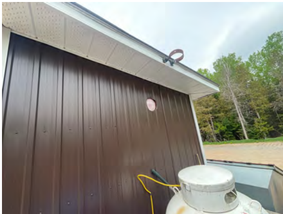
Raglan Transfer Station - B201008
