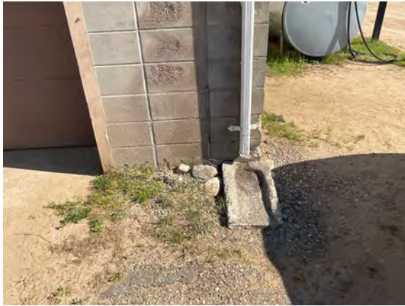
Quadville Public Works Garage - B301005
