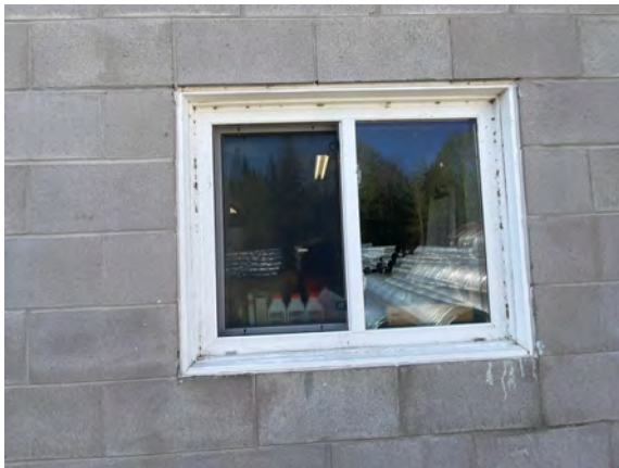
Quadville Public Works Garage - B202001
