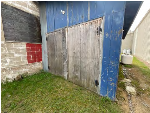
Palmer Fire Hall 1 - C102025
