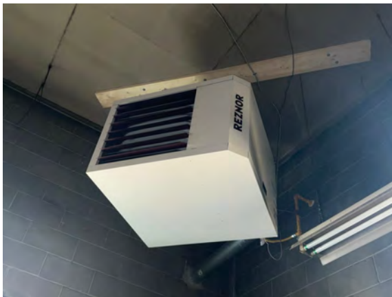
Palmer Public Works Garage - D302004
