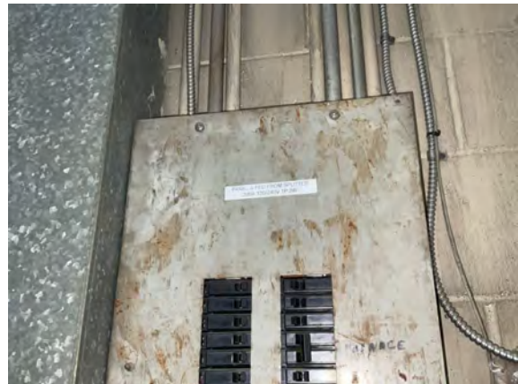
Palmer Public Works Garage - D502001
