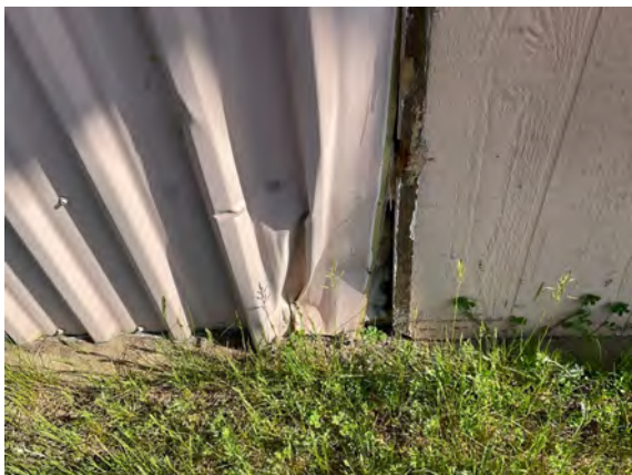
Quadville Public Works Garage - B201024
