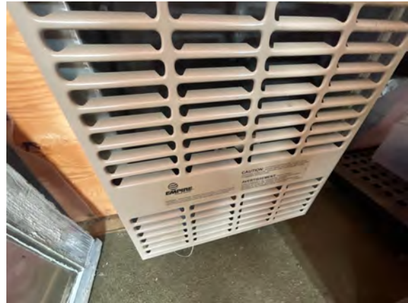
Raglan Transfer Station - D302004
