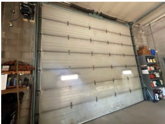
Quadville Public Works Garage - B203022
