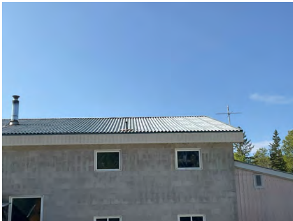
Quadville Public Works Garage - B301028
