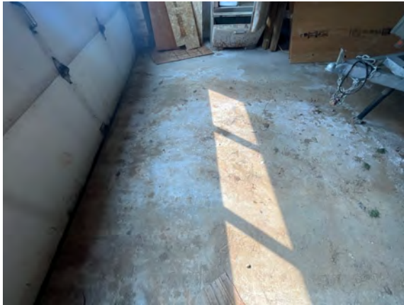
Palmer Storage Shed - A103001
