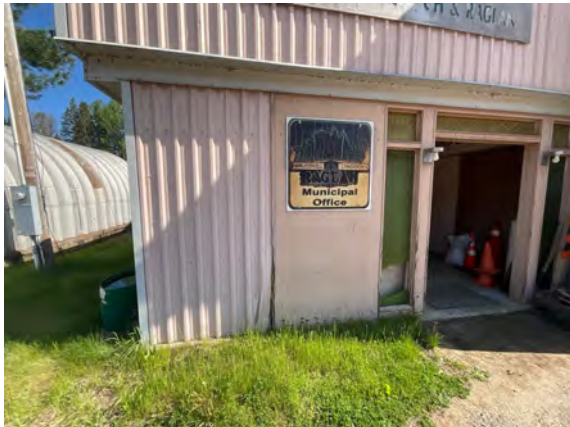
Quadville Public Works Garage - B201024
