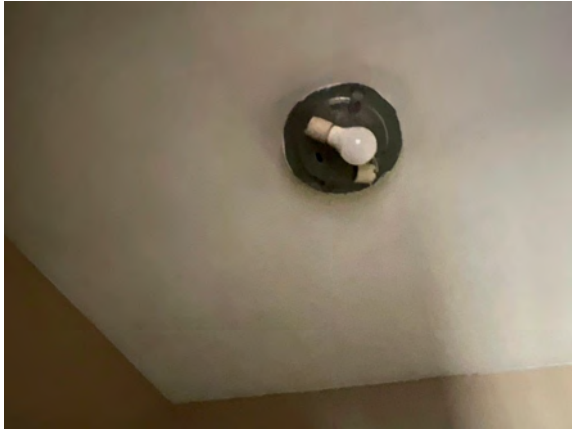
Quadville Public Works Garage - D502002
