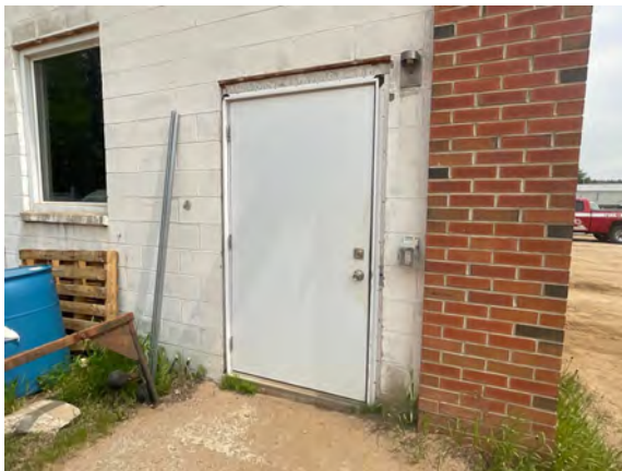
Palmer Public Works Garage - B203023
