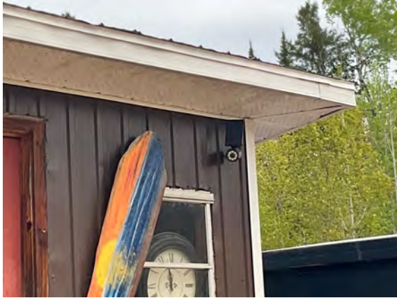
Raglan Transfer Station - G403099
