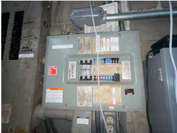
Palmer Public Works Garage - D501031
