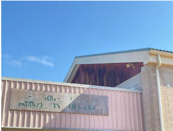
Quadville Public Works Garage - C103021
