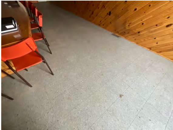
Palmer Fire Hall 1 - C302023
