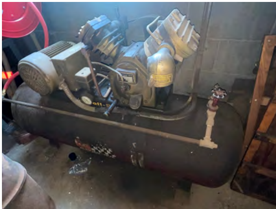
Palmer Public Works Garage - D209005
