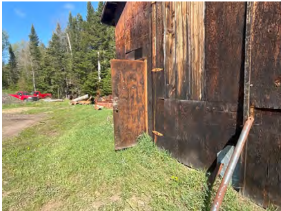
Storage Building - Quadeville - C102022
