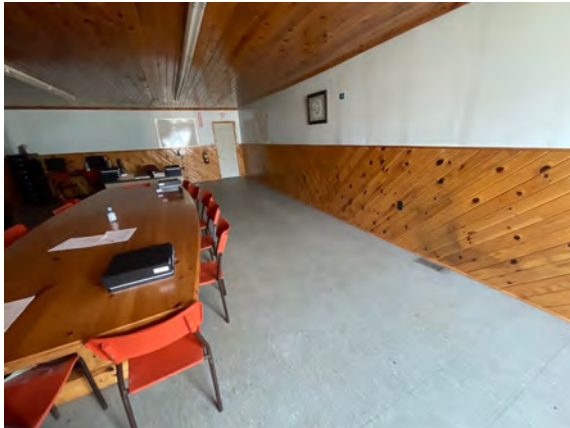
Palmer Fire Hall 1 - C301005
