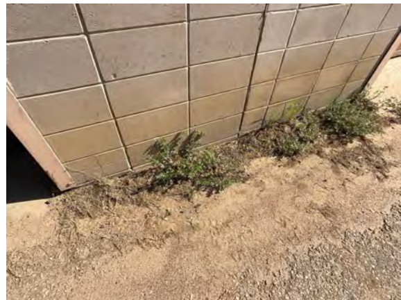
Quadville Public Works Garage - B201021
