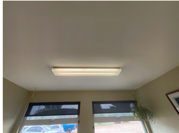
Township Office - C303006
