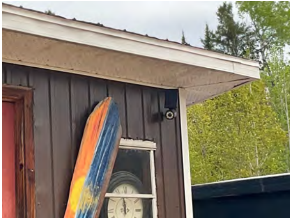
Raglan Transfer Station - B301028
