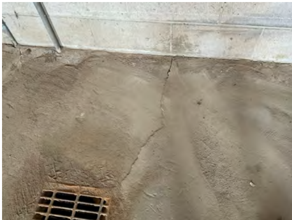
Quadville Public Works Garage - A103001
