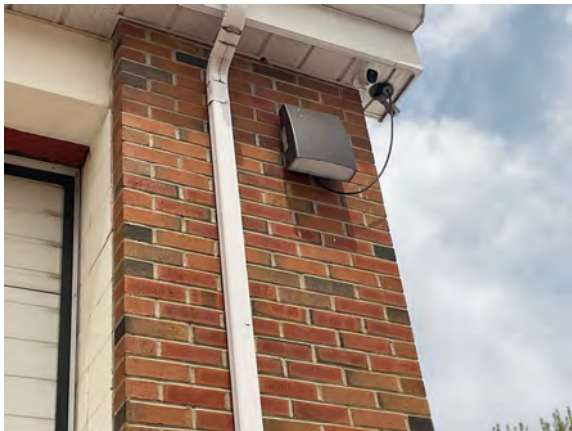
Palmer Public Works Garage - B301005
