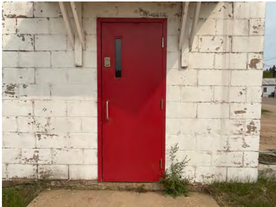
Palmer Fire Hall 1 - B203023
