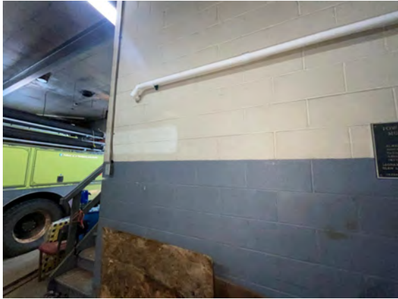
Palmer Public Works Garage - C303005
