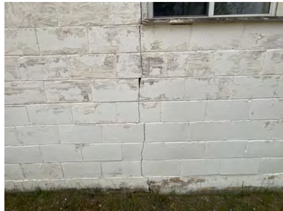
Palmer Fire Hall 1 - B201021
