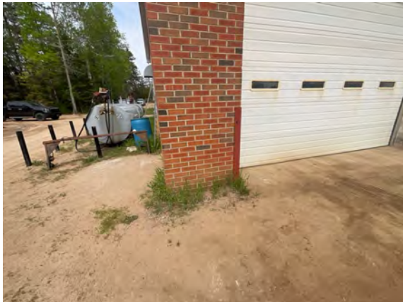
Palmer Public Works Garage - B201021
