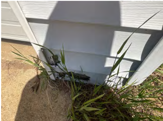
Brudenell Fire Hall #4 - B201025
