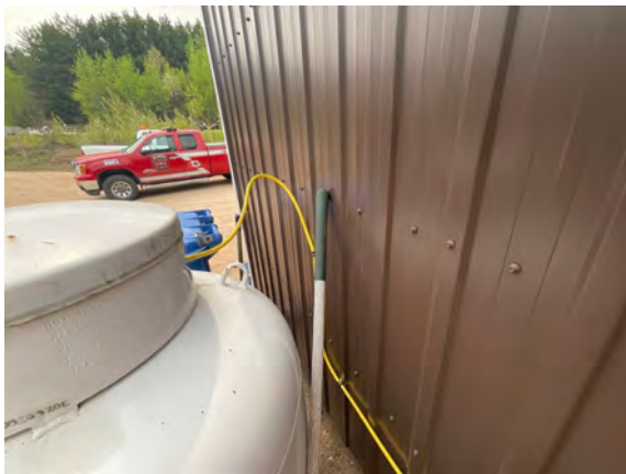
Raglan Transfer Station - B201024
