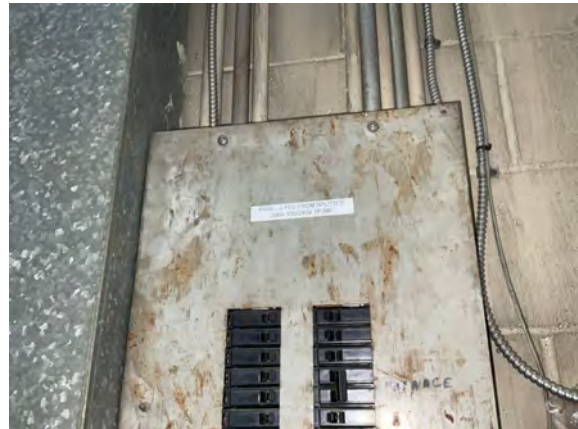
Palmer Public Works Garage - D501031
