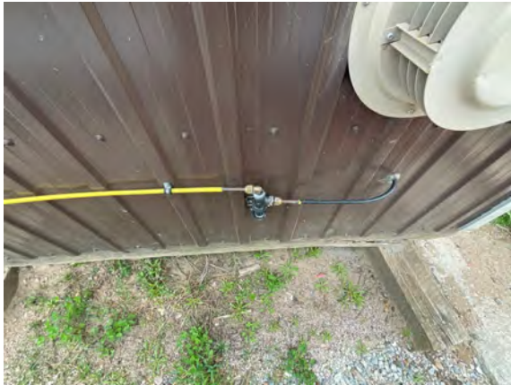
Raglan Transfer Station - D301002
