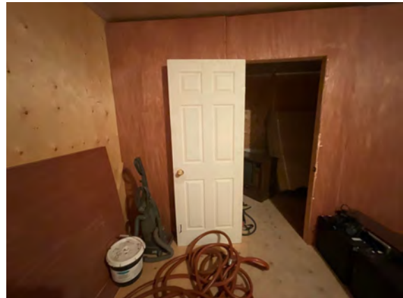
Palmer Fire Hall 1 - C102022
