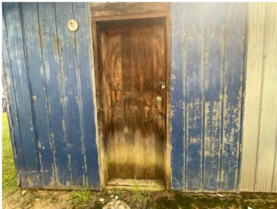
Palmer Fire Hall 1 - B203024
