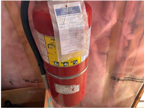
Raglan Transfer Station - D403002
