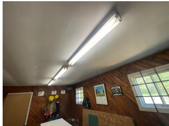
Brudenell Fire Hall #4 - D502002
