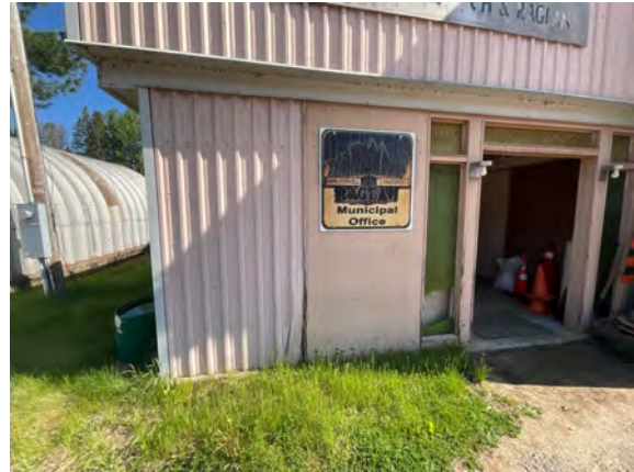
Quadville Public Works Garage - C103021
