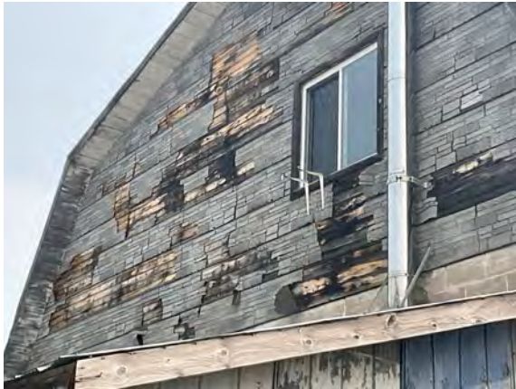
Palmer Fire Hall 1 - B201026
