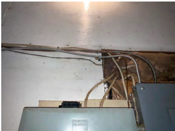
Brudenell Fire Hall #4 - D502001
