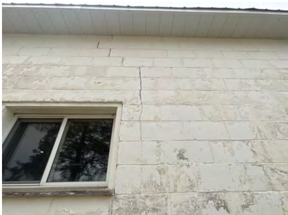
Palmer Fire Hall 1 - B201021
