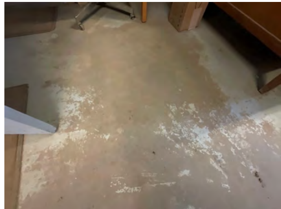
Quadville Public Works Garage - A103001
