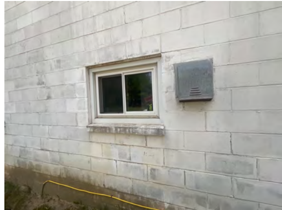
Palmer Public Works Garage - B201010
