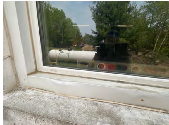
Palmer Public Works Garage - B202001
