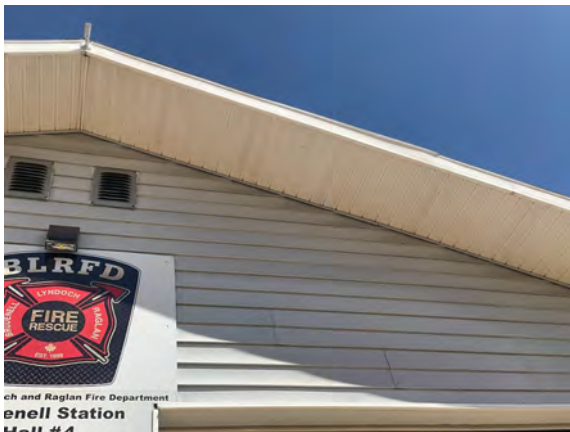
Brudenell Fire Hall #4 - B201008
