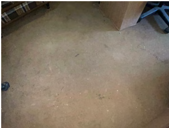
Palmer Public Works Garage - A103001
