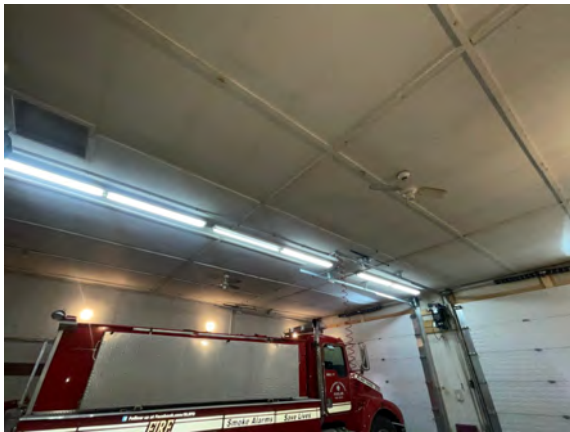
Brudenell Fire Hall #4 - B103001
