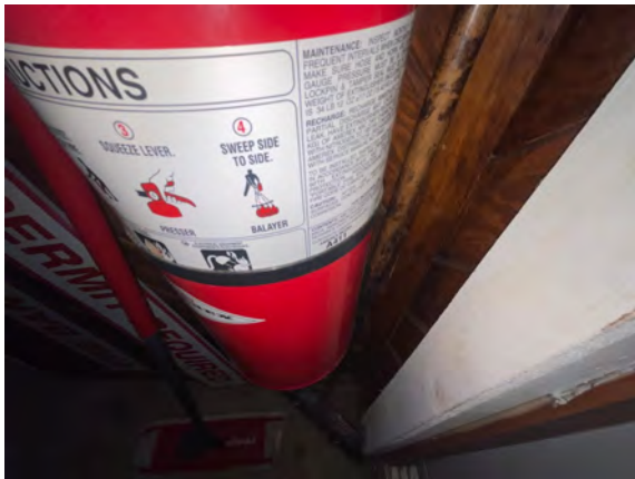
Brudenell Fire Hall #4 - D403002
