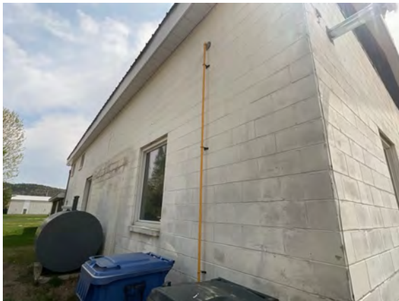
Palmer Public Works Garage - D301001
