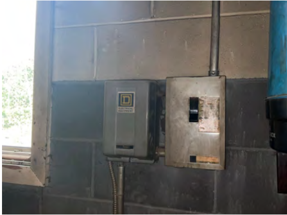
Palmer Public Works Garage - D501031
