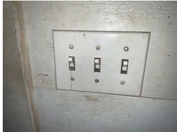
Brudenell Fire Hall #4 - D502001
