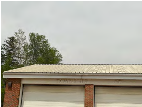
Palmer Public Works Garage - B301028
