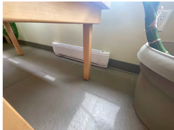
Township Office - C302023
