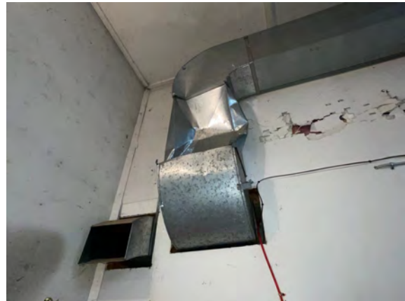
Brudenell Fire Hall #4 - D304001
