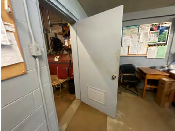
Quadville Public Works Garage - C102022
