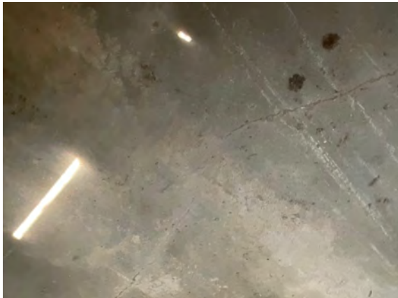
Palmer Public Works Garage - C302007
