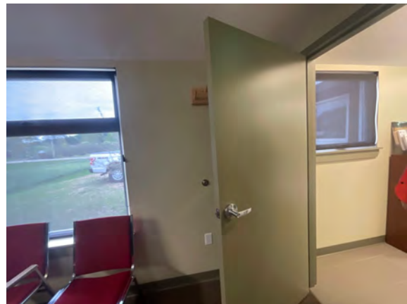
Township Office - C102022
