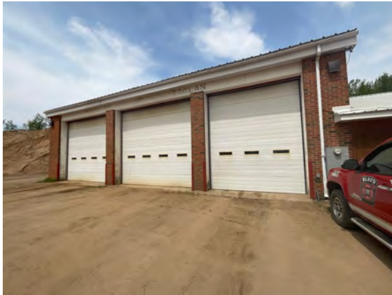
Palmer Public Works Garage - B203022
