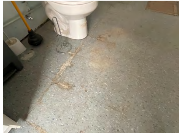
Palmer Fire Hall 1 - C302023
