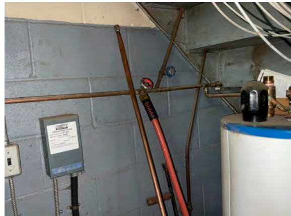
Palmer Public Works Garage - D202001
