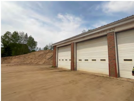
Palmer Public Works Garage - G201025
