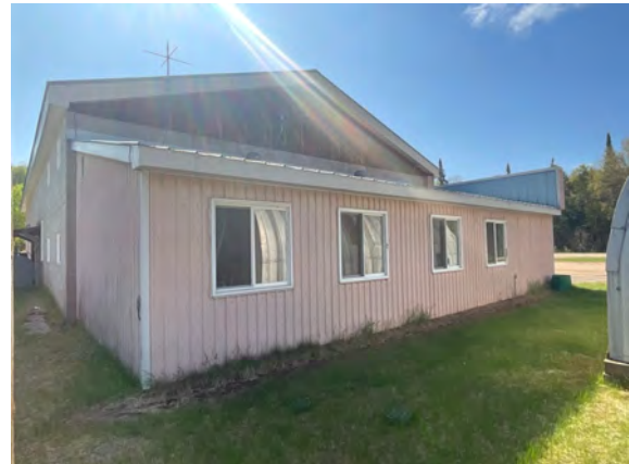
Quadville Public Works Garage - B201024
