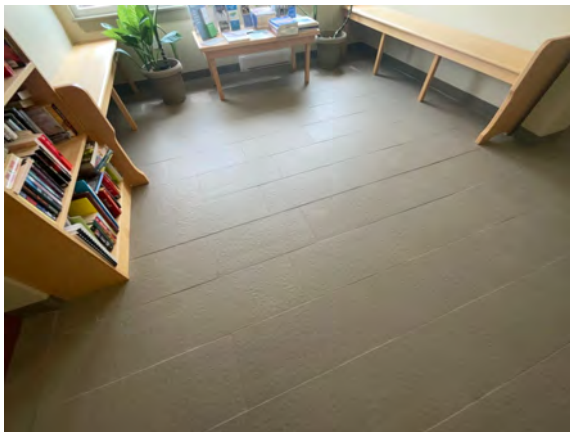
Township Office - C302023
