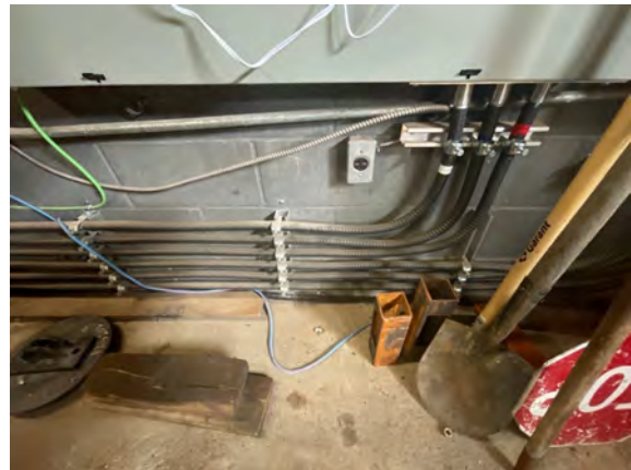
Palmer Public Works Garage - G401011
