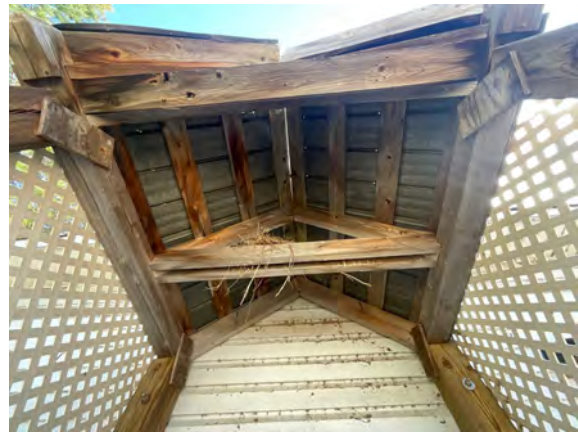
Quadville Fire Hall #3 - F101099
