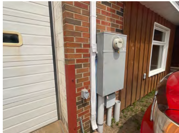
Palmer Public Works Garage - B301005
