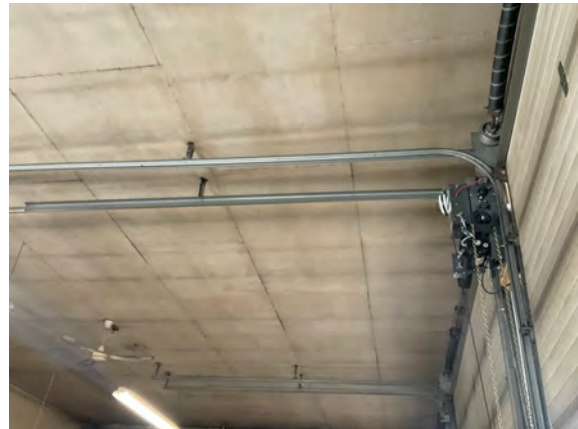
Palmer Public Works Garage - C303005
