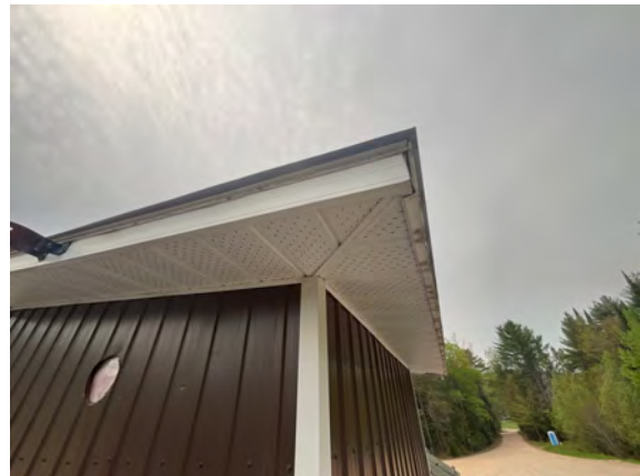
Raglan Transfer Station - B201008
