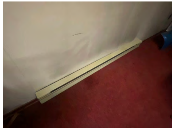
Quadville Public Works Garage - C302005
