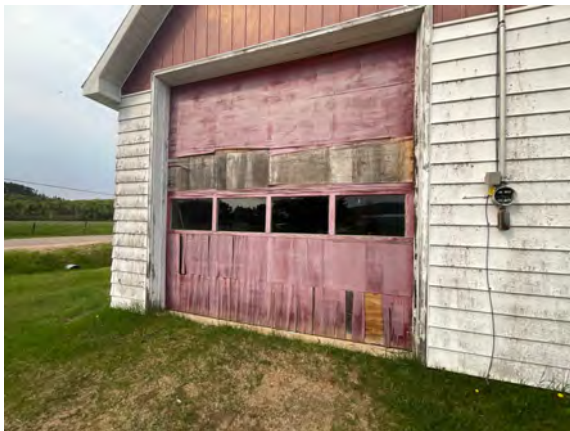
Palmer Storage Shed - C102005
