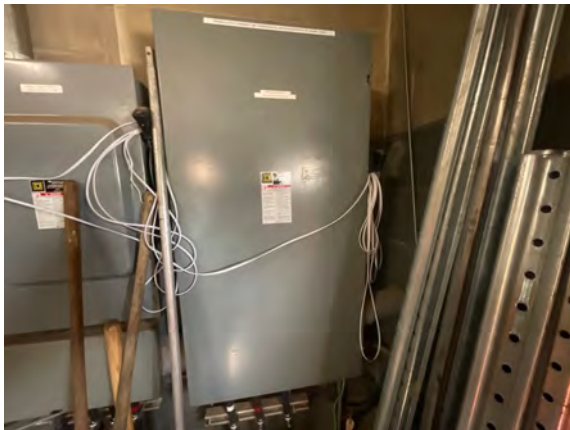
Palmer Public Works Garage - D501025
