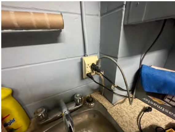
Quadville Public Works Garage - C301005
