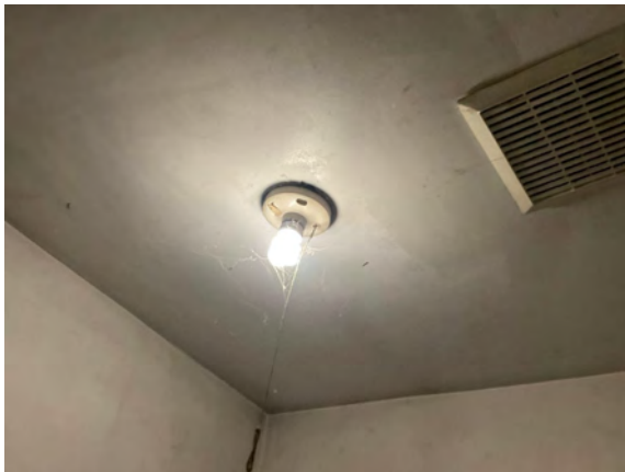
Brudenell Fire Hall #4 - D502002
