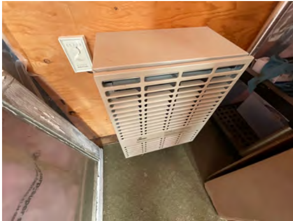
Raglan Transfer Station - D302004
