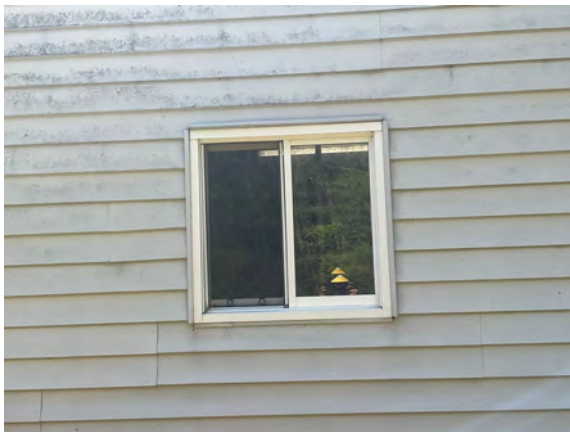
Brudenell Fire Hall #4 - B202001
