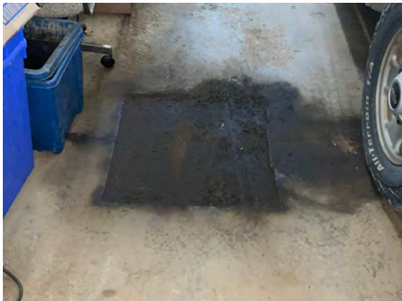
Palmer Public Works Garage - A103001
