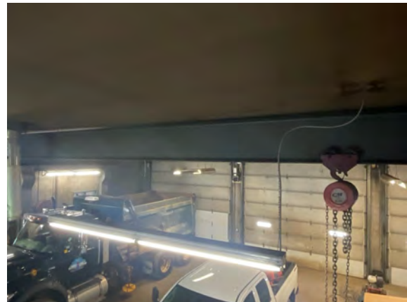
Quadville Public Works Garage - B103001
