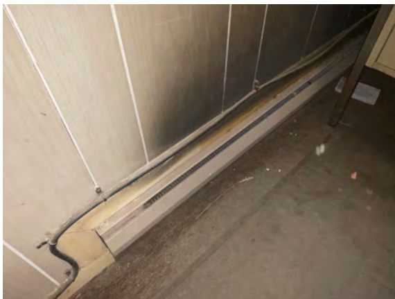
Palmer Public Works Garage - C301022
