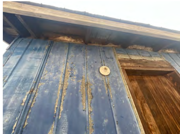
Palmer Fire Hall 1 - B201024
