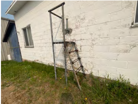
Palmer Fire Hall 1 - C201002
