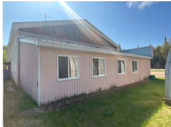
Quadville Public Works Garage - B202001
