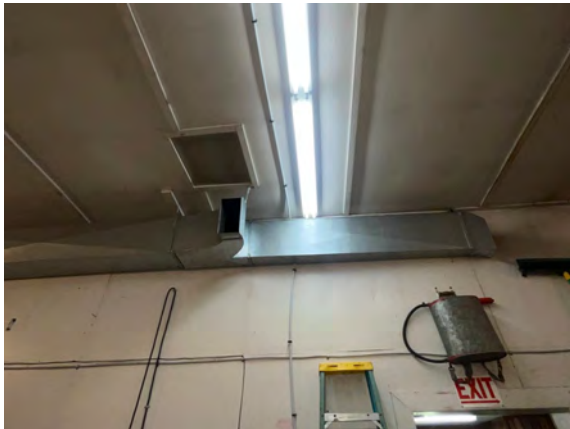
Brudenell Fire Hall #4 - D304001
