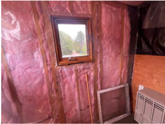
Raglan Transfer Station - B202001
