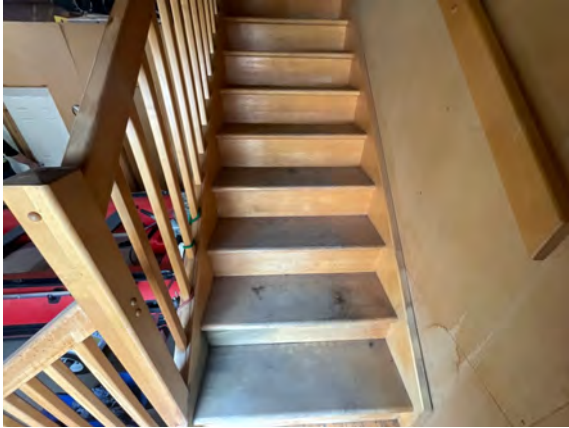
Palmer Fire Hall 1 - C201001
