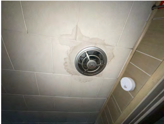
Palmer Public Works Garage - D304033
