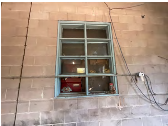
Quadville Public Works Garage - C101005
