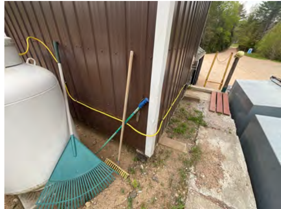
Raglan Transfer Station - D301002
