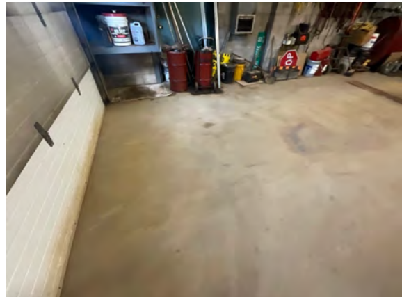
Quadville Public Works Garage - C302007
