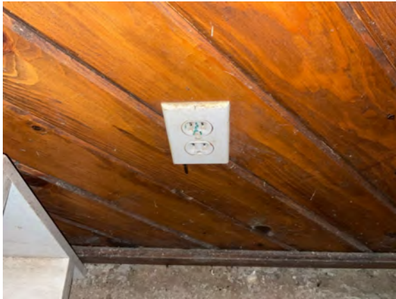
Brudenell Fire Hall #4 - D502001
