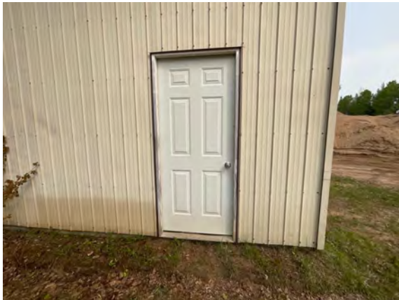
Palmer Storage Shed 2 - C102021
