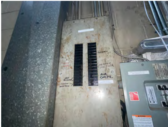
Palmer Public Works Garage - D501031
