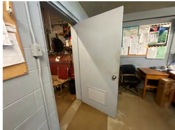
Quadville Public Works Garage - C301005
