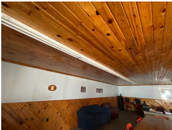
Palmer Fire Hall 1 - C301022
