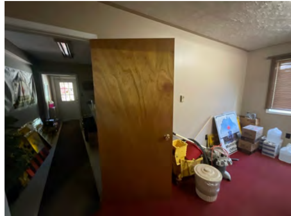
Quadville Public Works Garage - C102022
