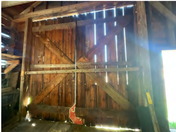
Storage Building - Quadeville - C102025
