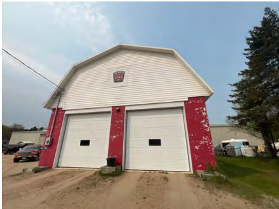
Palmer Fire Hall 1 - B203022
