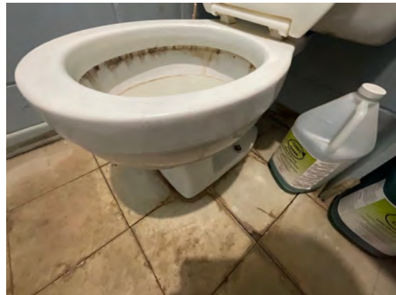
Quadville Public Works Garage - D201001
