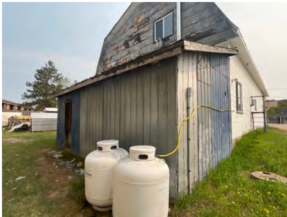
Palmer Fire Hall 1 - B201024
