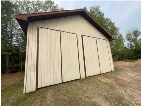
Palmer Storage Shed 2 - C102024
