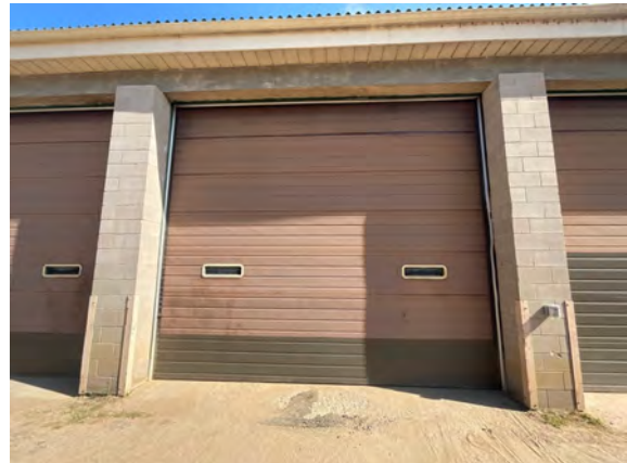
Quadville Public Works Garage - B203022
