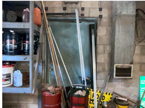
Quadville Public Works Garage - B203023
