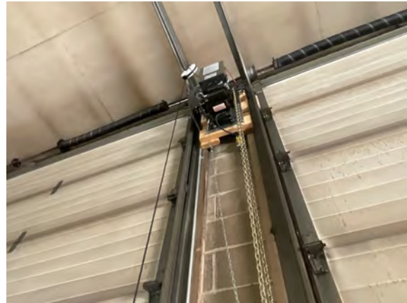
Palmer Public Works Garage - B203022
