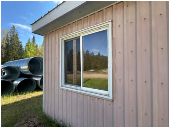
Quadville Public Works Garage - B202001
