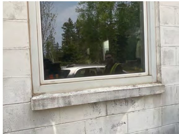
Palmer Public Works Garage - B202001
