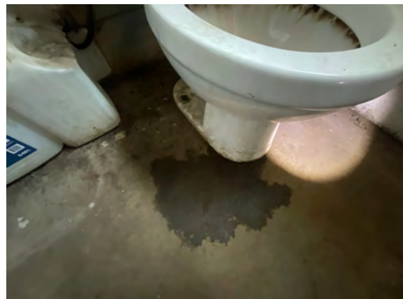
Quadville Public Works Garage - D201001
