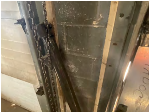
Palmer Public Works Garage - B203022
