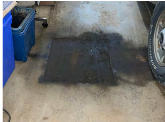
Palmer Public Works Garage - C302007
