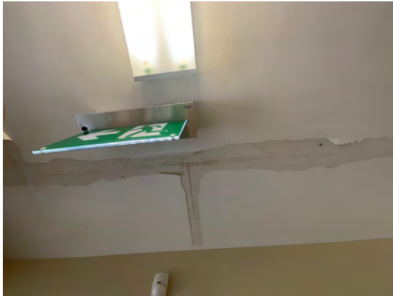
Township Office - C303006
